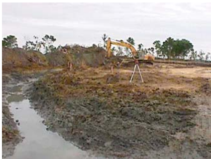
Figure 7: Equipment used to grade the site to specific elevations.
