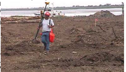
Figure 6: Grading stakes set by elevation survey (ATM, 2005b).
