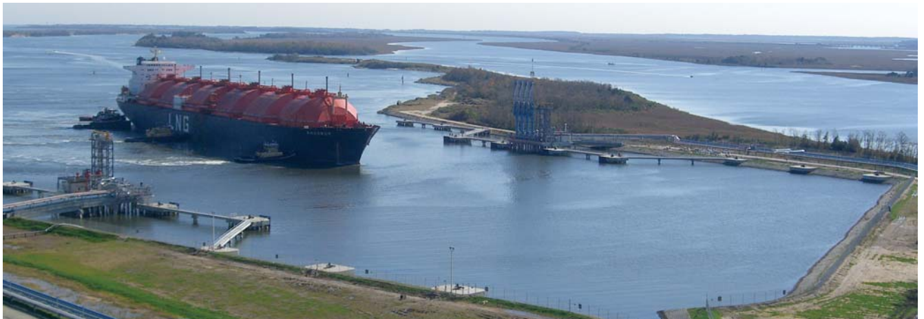
Figure 3: Entry of the first ship into the new LNG slip, February 2, 2006.
