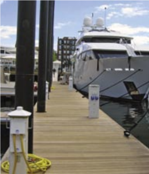
Close-up view of new docks at Forty 1° North. The original bulkheads and docks had deteriorated badly.
