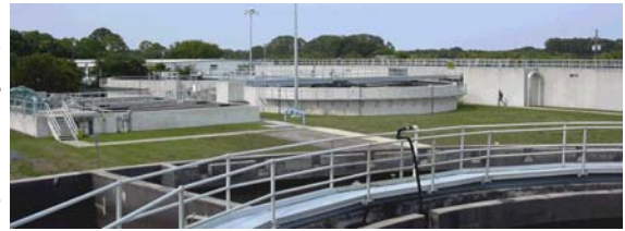
Atlantic Beach WWTP
