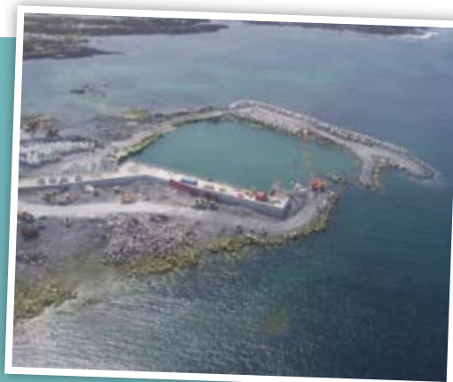
Caladh Mór under construction
