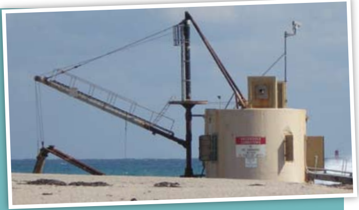
Fixed inlet bypassing plant at Palm Beach's Lake Worth Inlet
