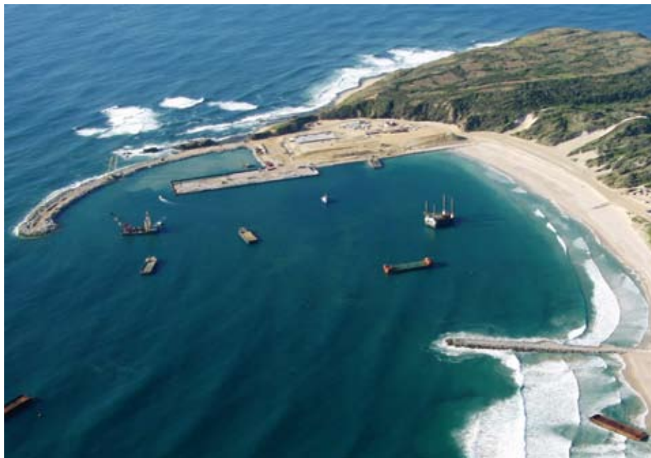
Work under way on Port d'Ehoala in September 2008
